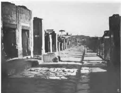
Fig. 406.—Specimen of the pavement of Roman roads and streets. The Via dell' Abbondanza at Pompeii.
